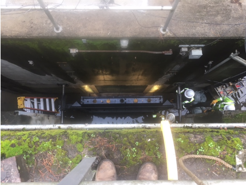
Figure 5. Overhead view of work area.
