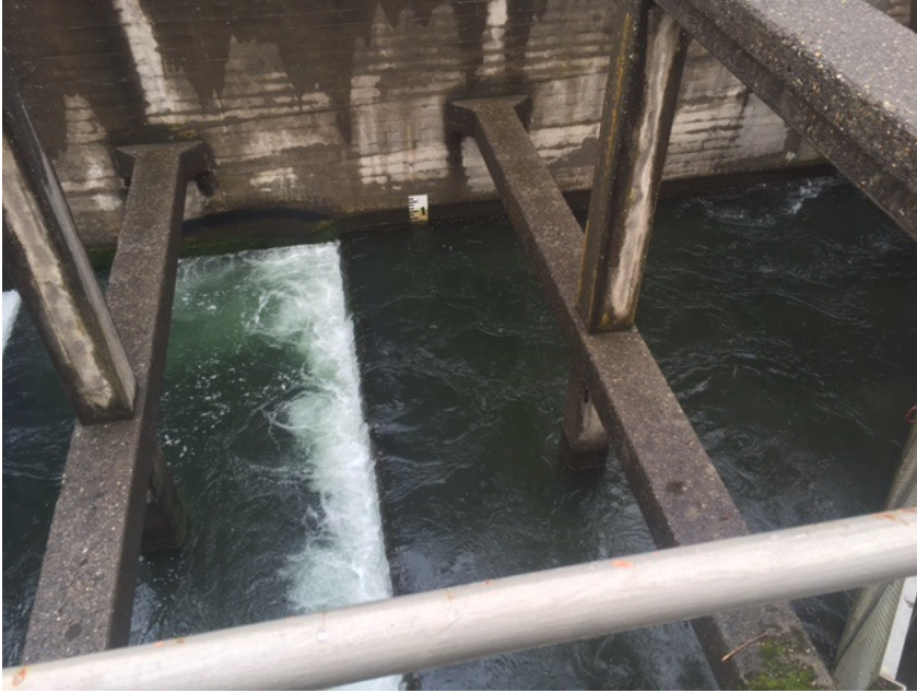
Figures 3. Water level at Cascades Island with FV 5-9 closed and UMT open. This is the level originally anticipated during the work period.
